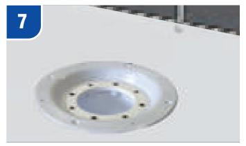
Also ensure that the flange on the trap body is level with, or slightly below the DEC.
