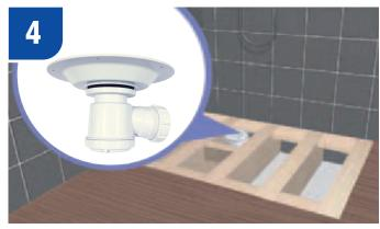
Connect the trap body to your outlet pipework, position between joists and centrally beneath the hole in the DEC.
